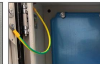
Grounding screw More aesthetically pleasing and safer
